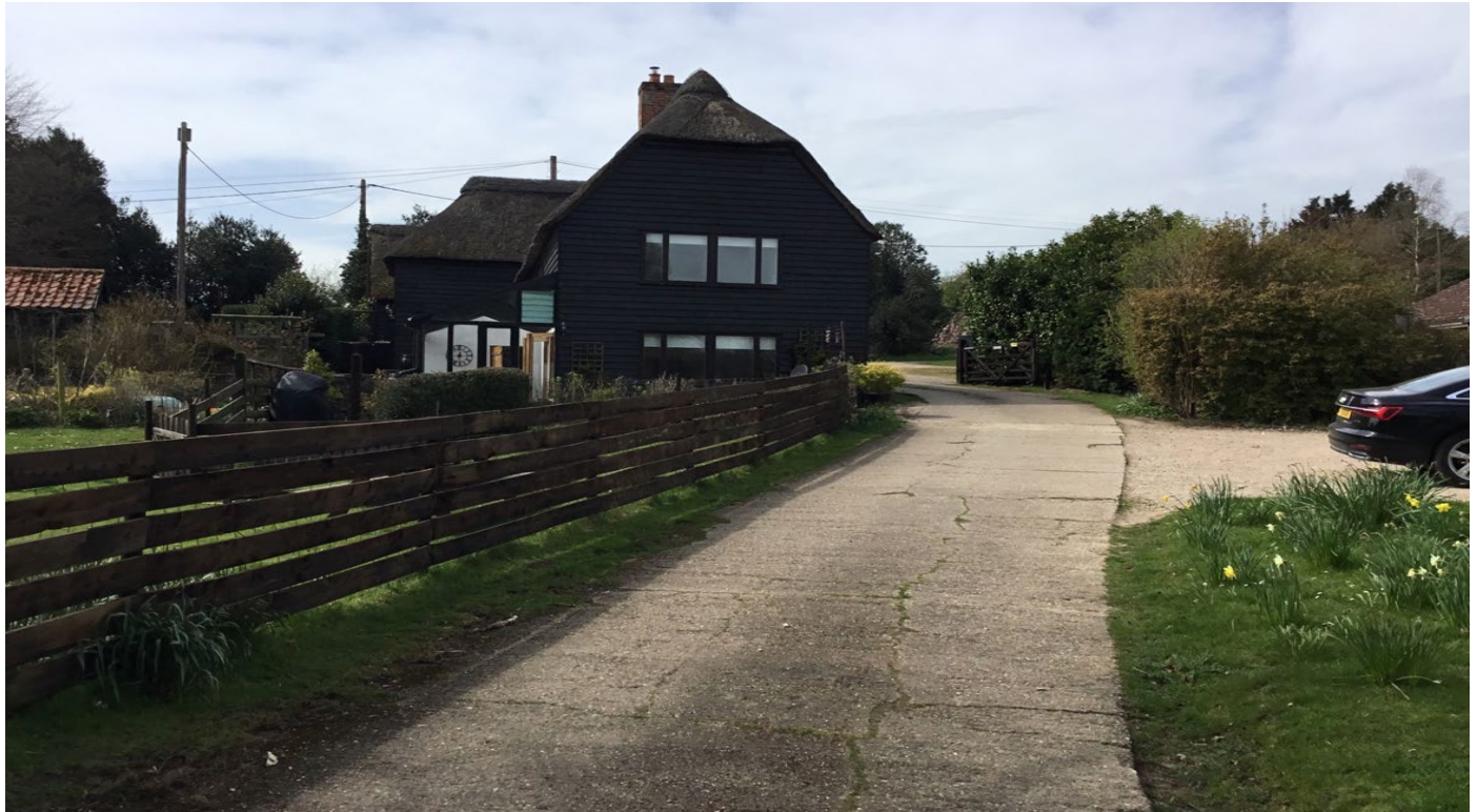
Access from the main highway to the rear of Marshes (left)
